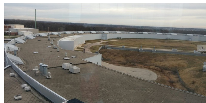
Huge circular Advanced Photon Source building where xrays are used to illuminate chemical reactions and molecules at the nanoscale level
